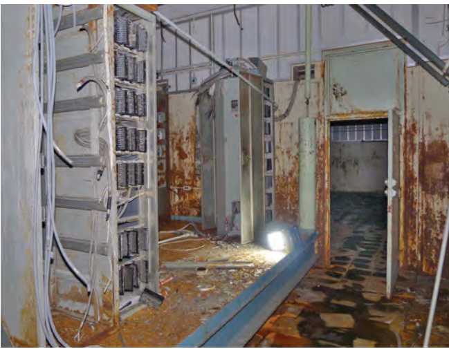
The crypto room, showing racks of communications equipment mounted on a shock isolated platform and the LAUT (Launch Area Utility Tunnel).
